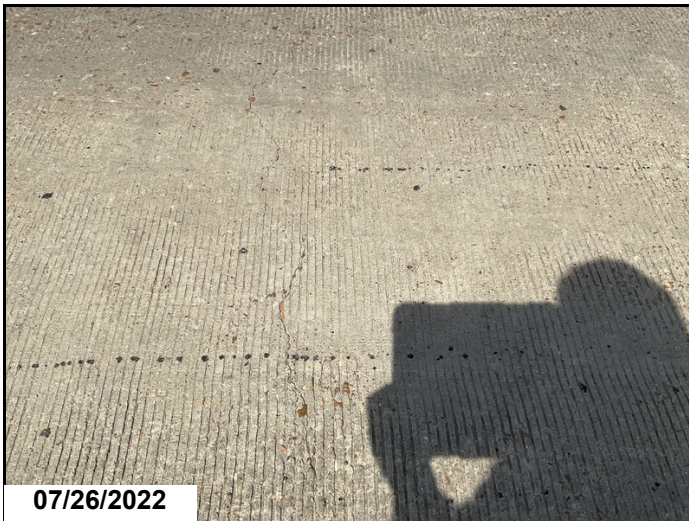
Typical transverse crack in approach slab
