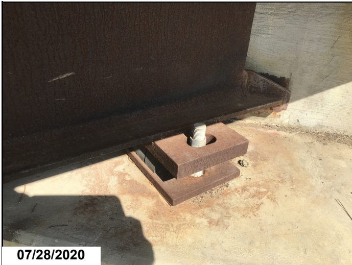
Abutment #2 typical missing bearing nut.
