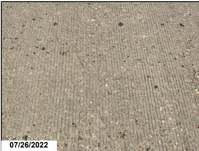
Typical transverse deck crack
